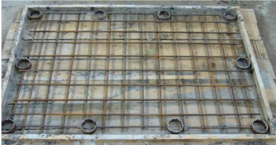
Figure 3. Reinforcement in slabs
