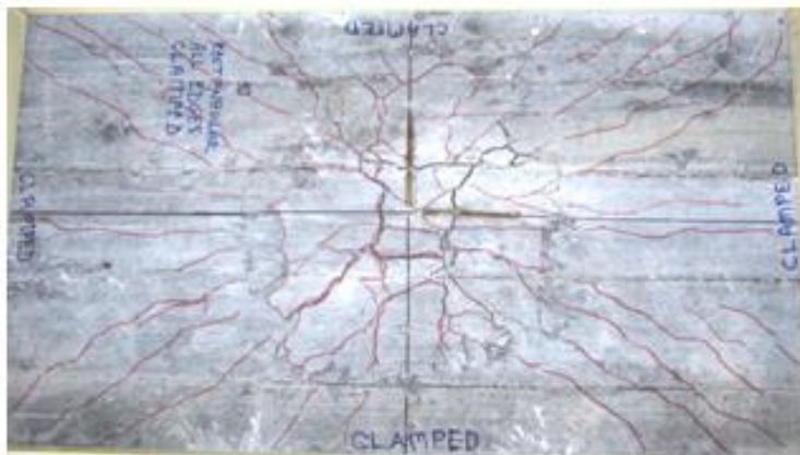
Figure 10. Failure pattern of AD4 slab
