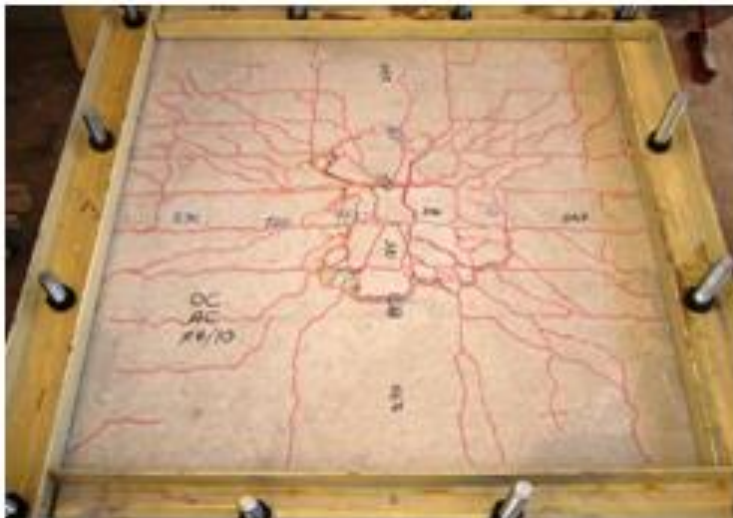
Figure 18. Failure pattern of AGB4 slab
