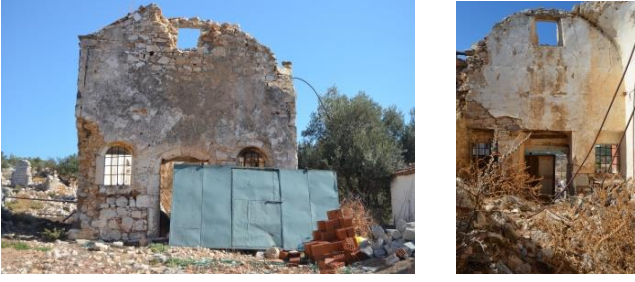
Figure 4. A ruined church building, Izmir (Olğun and Yörür, 2020)
