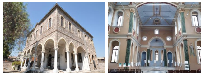
Figure 3. Ayavukla Church under conservation, Izmir (URL 2; Personal archive, 2018)
