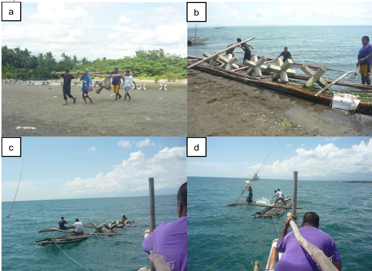
Figure 3. Deployment of ARs at Barangay Baguingin, Tigbauan, Iloilo, Philippines: (a) ARs were carried by municipal fisherfolks to the shoreline; (b) ARs were loaded to bamboo raft; (c) ARs were brought to the desired area of deployment; and (d) ARs were manually pushed to the water (Photo taken from Ariel S. Tentia, Tigbauan Municipal Bantay Dagat Member).
