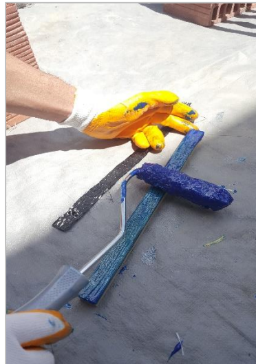
Figure 1. Wrapping process of wooden beams with FRP.
