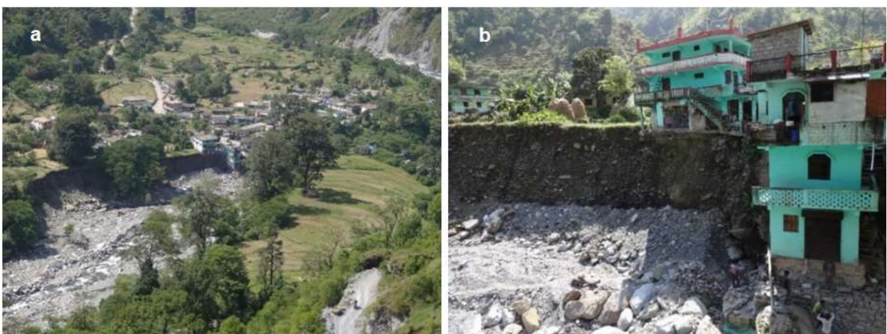
Fig. 14. View of eroded terrace with houses in vulnerable state on the left bank of Barar Gad; (a) panoramic view and (b) close view
