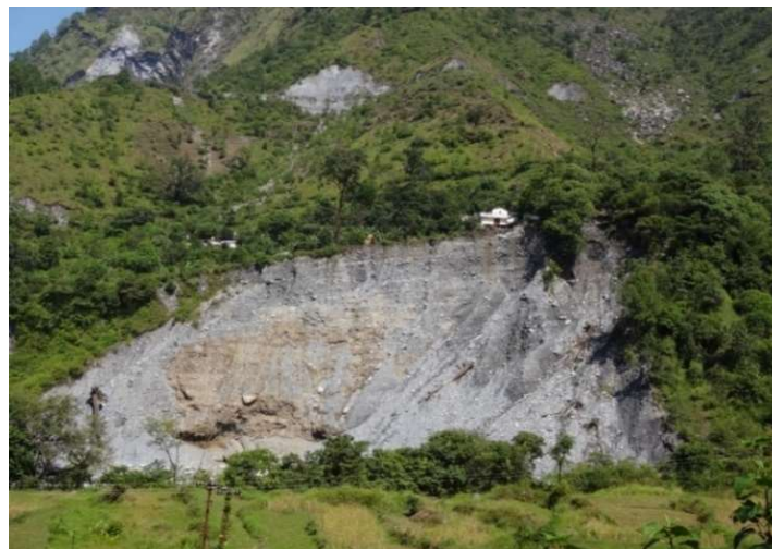
Fig. 13. Severally damaged a house in Khetali Village located in close proximity to eroded terrace cut that was eroded by Barar Gad
