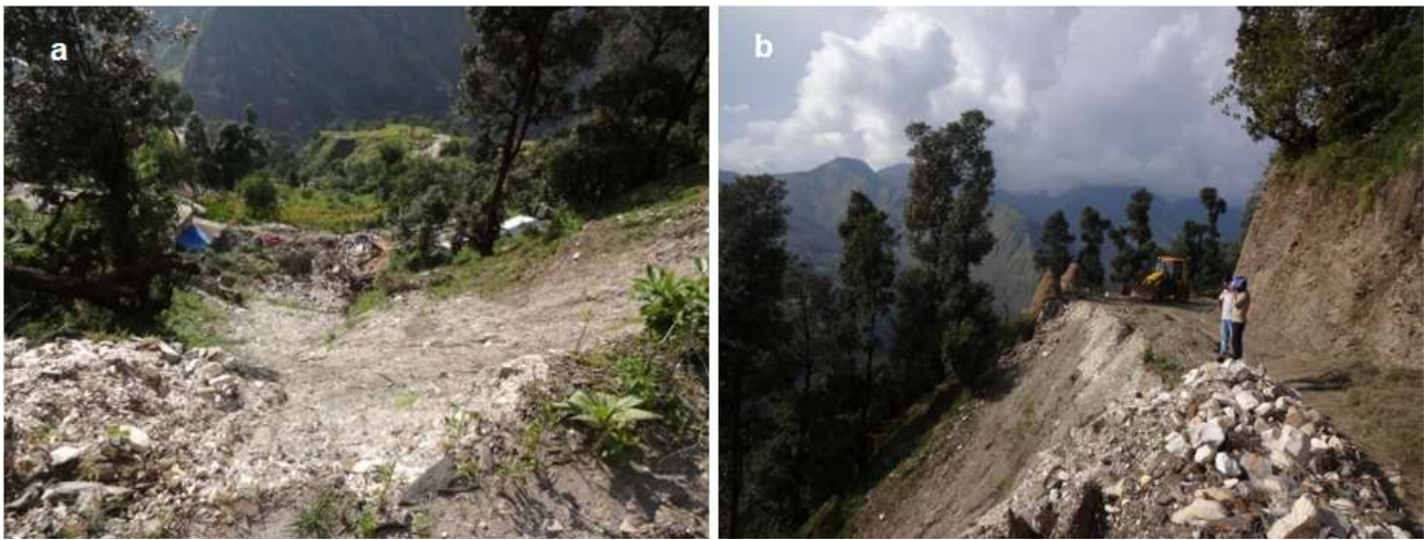
Fig. 12. Slope failure at Gaila Malla Tok in Pattharkot Village; (a) failure slope above destroyed house (b) damaged portion of under construction road
