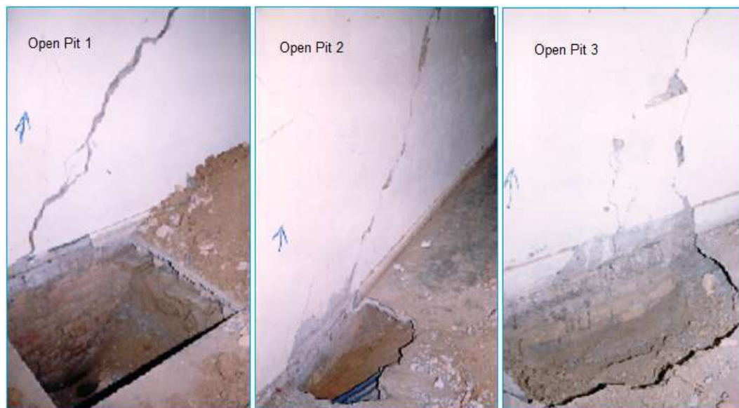
Fig. 7. Open pit settlement behavior of subsurface soil
