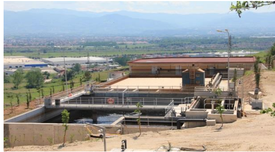
Figure 8. Landfill Leachate Water Treatment Facility General Appearance
