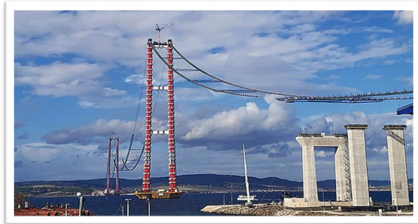
Photograph 2: 1915 Çanakkale Bridge Cat Trail Construction ( https://www.rehbercanakkale.com/1915-canakkale-koprusu-nde-kedi-yolu-da-bitiyor/6846/ )
