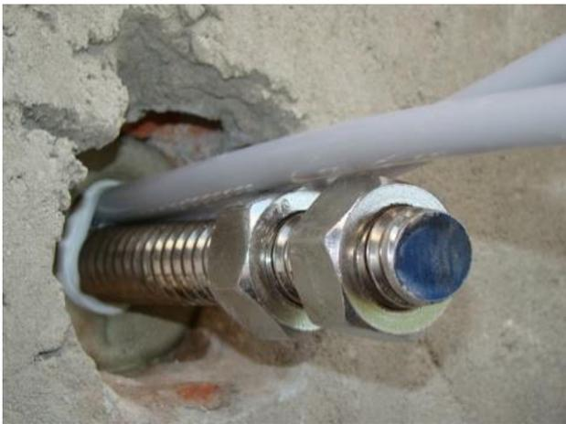
**Figure 43.** Anchorage in the masonry with the injection of grout limited by a sock.
