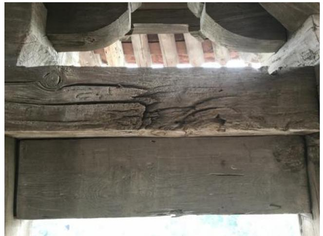
Figure 3. Damaged beam with knots
