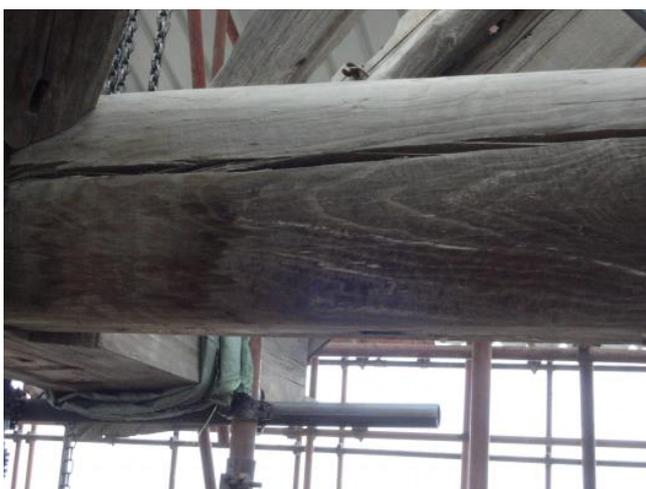
Figure 2. Cracks in square beam
