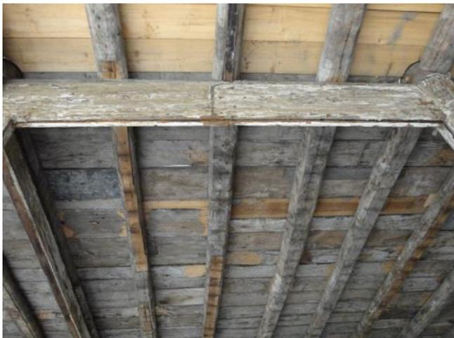
Figure 1. Cracks in square beam
