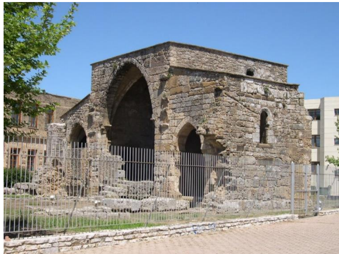
Figure 1. The vaults over the apse in Hagia Sophia, Andravida
