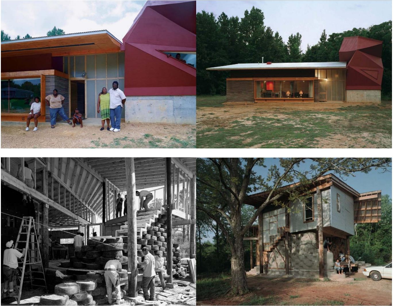
Figure 2-3. Shiles House, The Rural Studio, 2002. Students build the Shiles House which has a wall is made of old tires filled with dirt and covered with cement (Dean, 2005).
