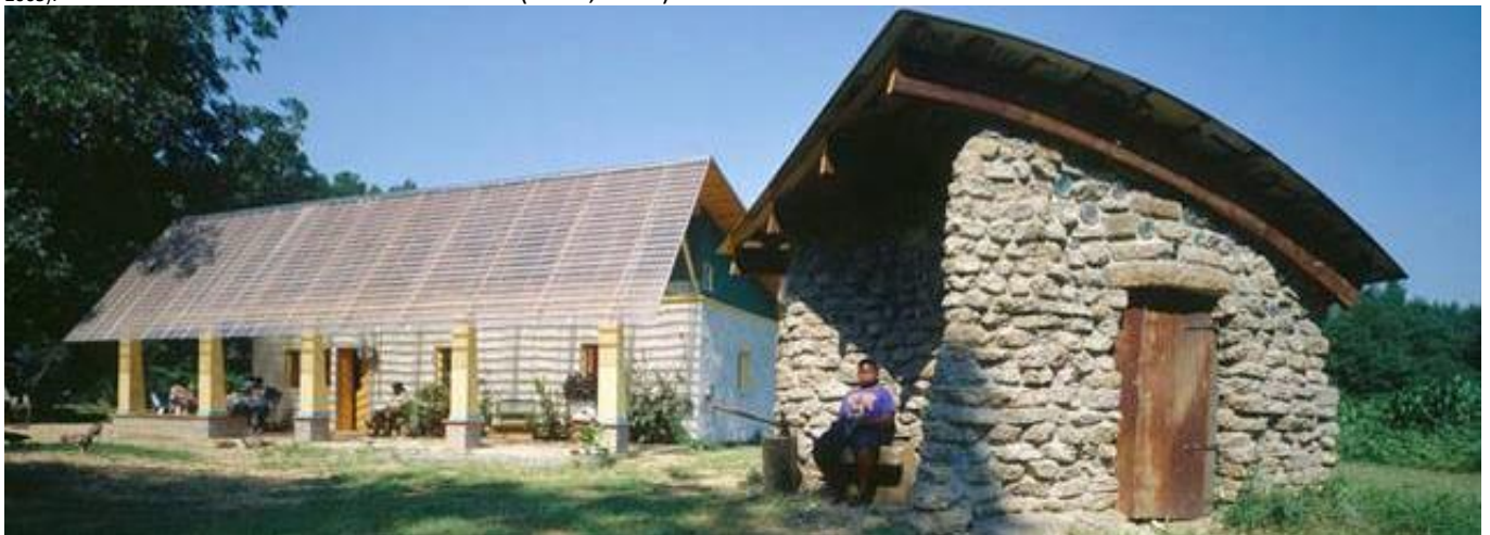
Figure 1. Smokehouse, The Rural Studio's first project, 1999. In the construction of the house, the walls of the main living part were built by hay bales, and stone with colored glass were used for the smokehouse (Dean, 2005).
