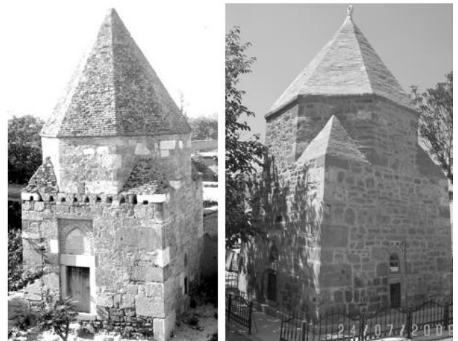
Figure 1. Fakih Dede Tomb north and south facade view
