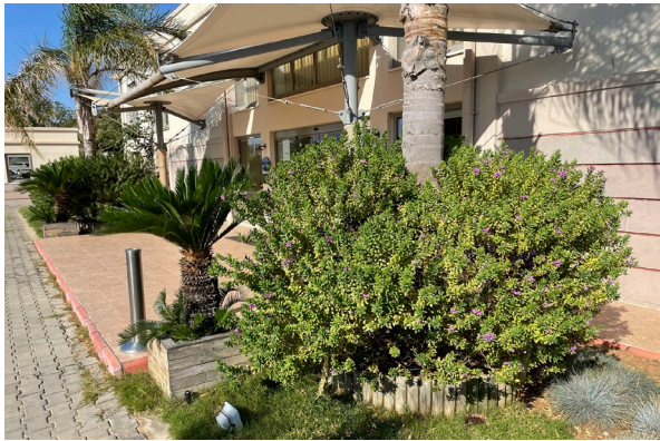
Figure 58. Front Section of the Administration Building, 2021 (Balik, 2021b)
