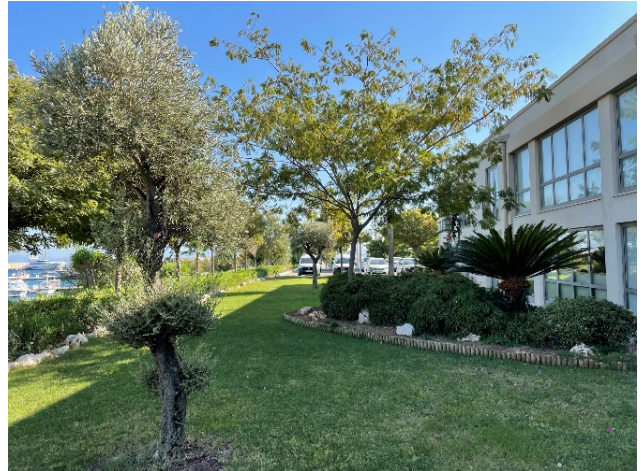
Figure 63. Administration Building: Rear Section No.3, 2021 (Balik, 2021b)
