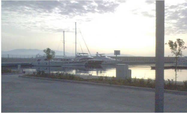
Figure 72. The Berth Area: Seaside Section, 2009 (Balik, 2021b)
