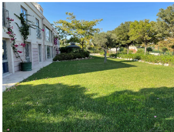
Figure 61. Administration Building: Rear Section No.1, 2021 (Balik, 2021b)
