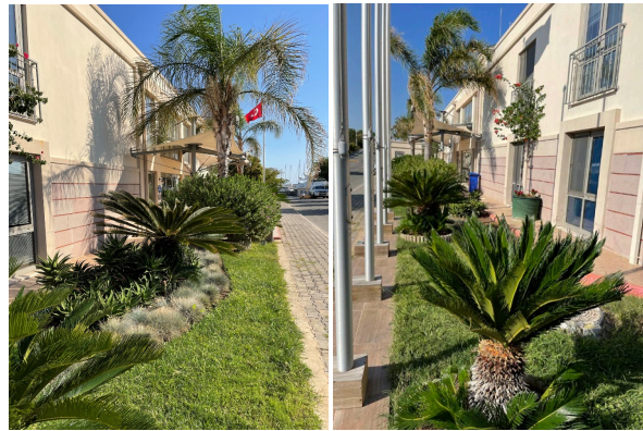
Figure 59. Front Section of the Administration Building, from Left and Right, 2021 (Balik, 2021b)
