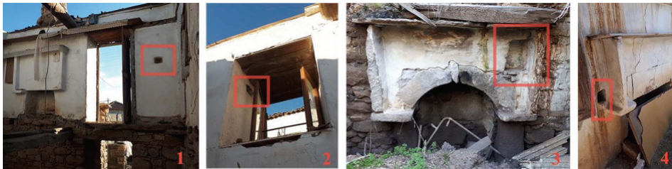
F. 13: 1: Small niche in fireplace wall but not next to fireplace in H1. 2: Small niche in window opening in H1. 3: Small niche under ocak başı in H10. 4: Small niche next to fireplace in H14. (Photos by Sarıbekiroğlu, 2017)
