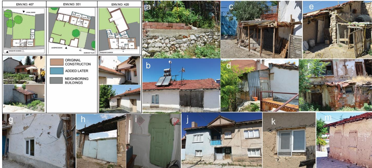
Figure 8. Problems encountered in buildings
