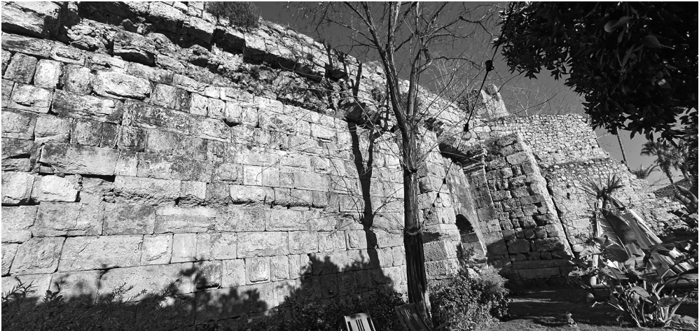
FIG. 16 Curtain wall and Gate. West façade (B. Varkivanç).
