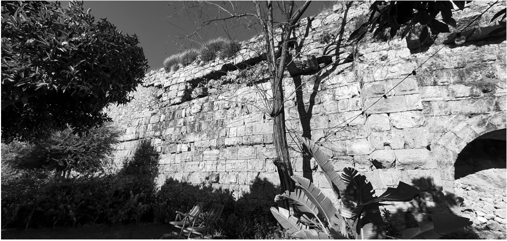
FIG. 15 Curtain wall and Gate. West façade (B. Varkivanç).
