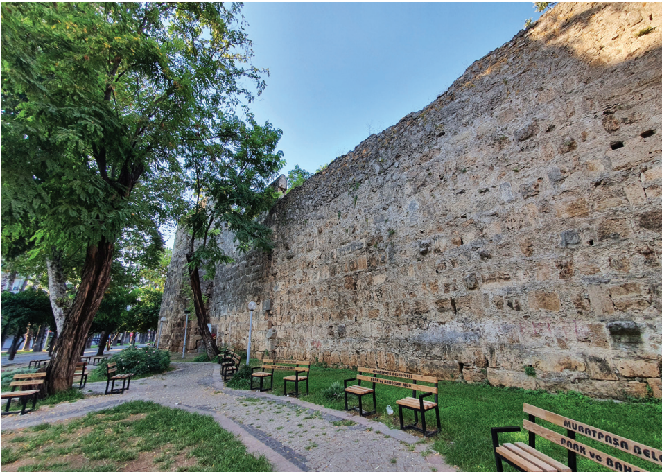
FIG. 19 Curtain wall. East façade (B. Varkıvanç).
