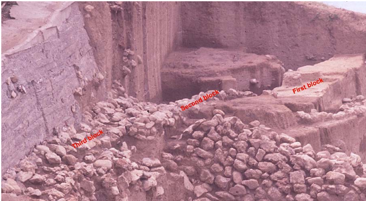
Fig. 7 Bakla Tepe phase BT IV 1 C, fortification wall with a saw-tooth pattern.
