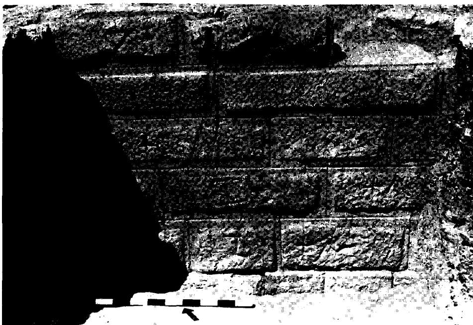
Fig. 28. Sector MMS-N, Lydian East Wall, sandstone masonry, looking northeast.
