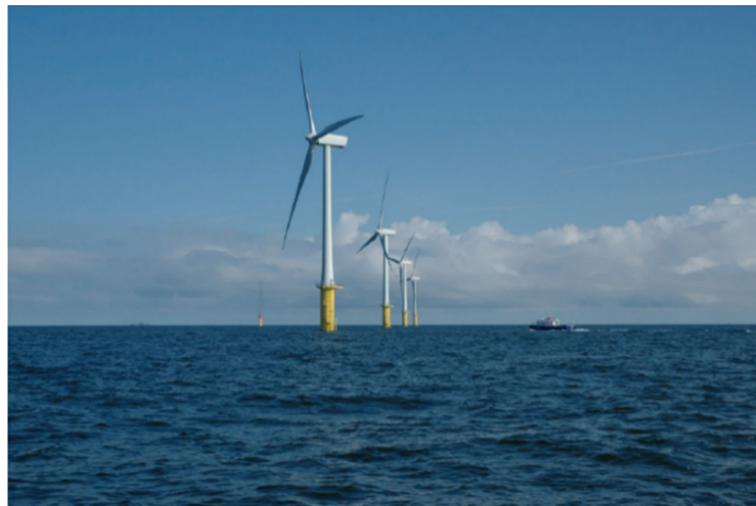
Figure 8. Vestas V80 - 2.0 offshore wind turbines of the North Hoyle wind farm (Hau, 2013).
