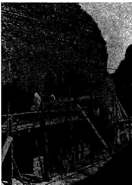
Fig. 2 — Gymnasium. Repair of west wall arches; Hall BE-H with swimming pool.
