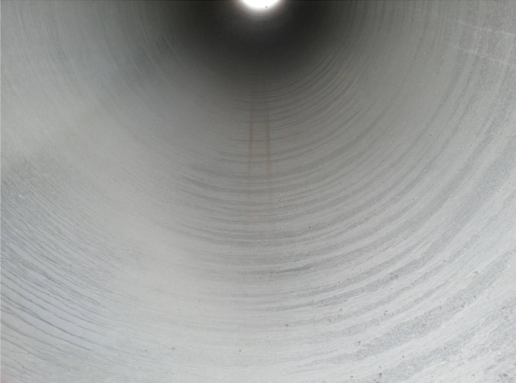
Figure 4: Interior concrete lining of the pipe from factory,[22]
