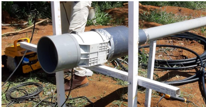
Figure 6. Blowing of ambient air inside the pipes using a fan.
