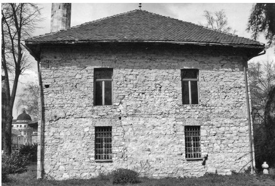
Figure 6. The rear elevation after the stucco removal (Photo by Edin Jahić)
