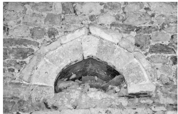
Figure 7. Uncovered arch over the original upper window (Photo by Edin Jahić)
