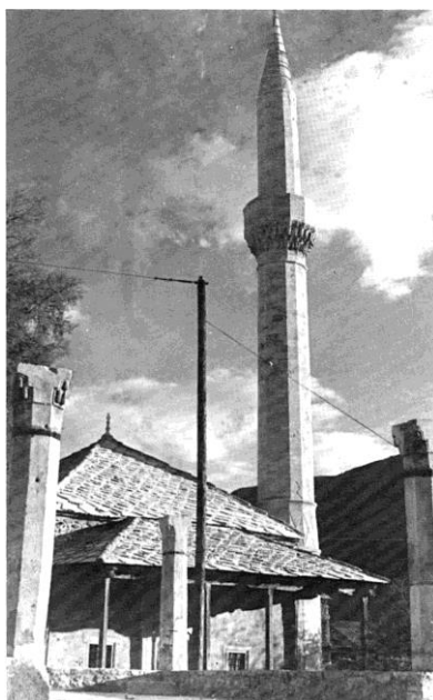
Figure 10. Roznamedži Ibrahim Efendi Mosque in Mostar. An example of mosque with pyramidal roof over the square prayer room and pitched roof over the porch. (Source: Hasandedić, 2005)
