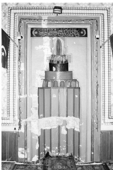
Figure 8. Mihrab during the research works (Photo by Edin Jahić)
