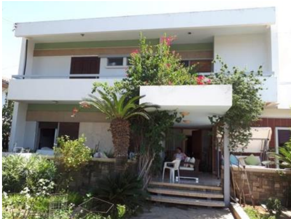
Figure 10 - A Façade of A modern house example from 60's in Güzelyurt (Authors, 2021).
