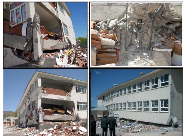
Figure 1.Çeltiksuyu Regional primary Education School Building
