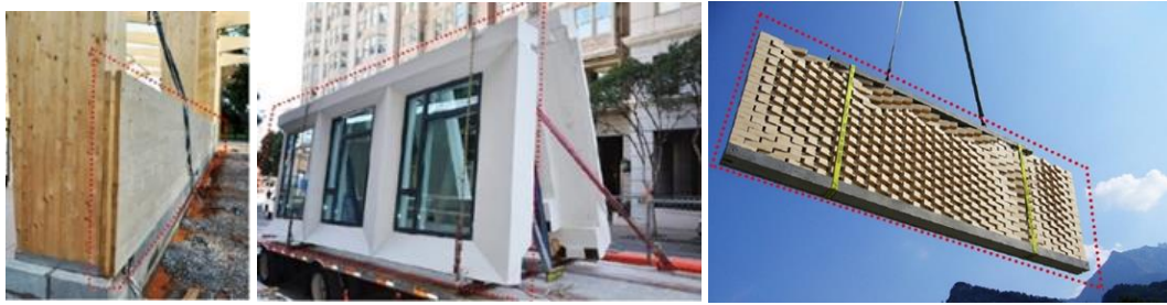
Figure 4. Examples of massive prefabricated facade panels based on wood, concrete, and terracotta (CLT; The Rockwell; Brick Research, 2022)
