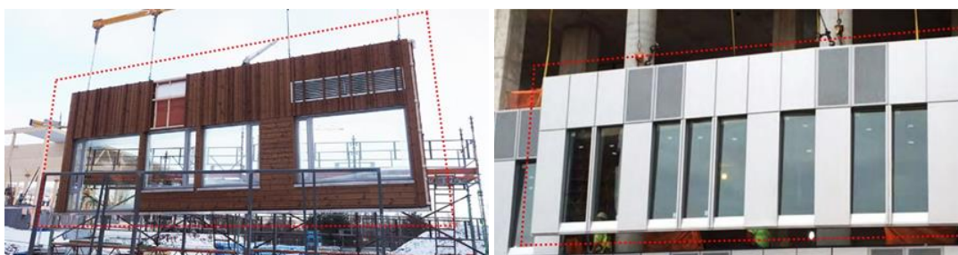
Figure 6. Examples of frame prefabricated facade panels based on wood and metal (Cornell Tech NYC; Jørn Hindklev, 2022)
