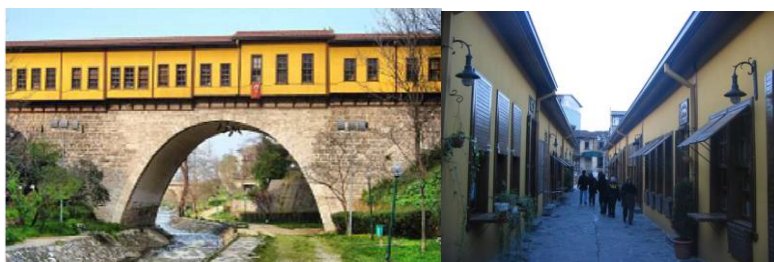
Fig10. The Irgandi Bridge (Source: www. google earth.com)
