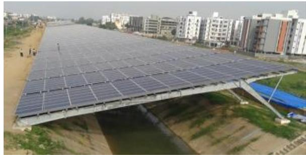
Fig. 4. The Canal-top Solar [6]
