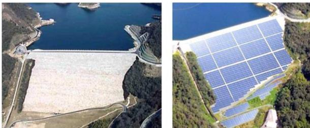
Fig. 2. The Surface SPP of a Dam [4]
