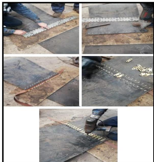
Figure 8. Images of the mechanical splicing application
