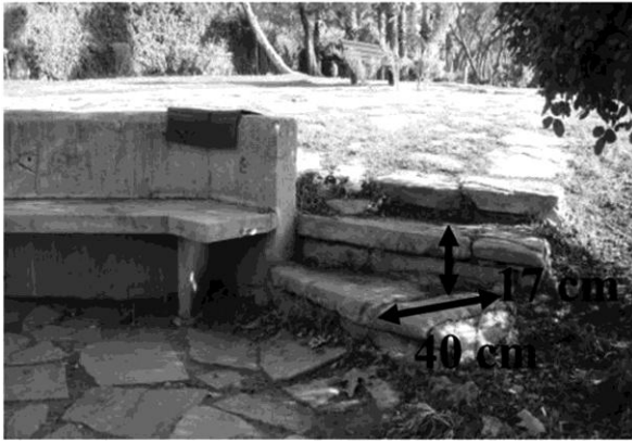
Figure 10. Entry stairs of Antalya Atatürk Culture Center and section of stairs (Original 2010)
