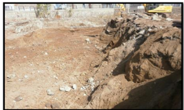
Figure 6. Phase1-Slope excavation in the field
