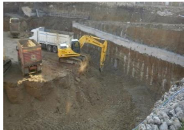
b) Phase 2-Excavation up to the anchor level at the site
