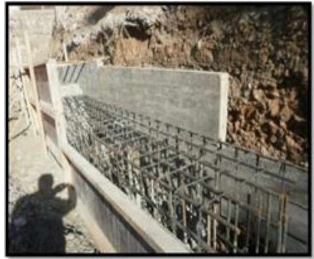
Figure 8. Phase 1 Capping beam construction
