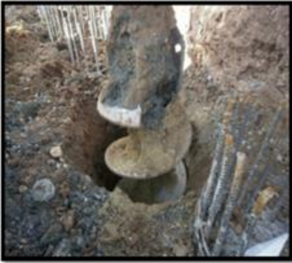
Figure 7. Phase 1 Bored pile construction
