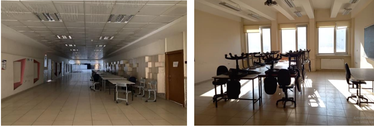
Figures 19 and 20. 304B interior view and recess corridor (Tohidi, 2020).
