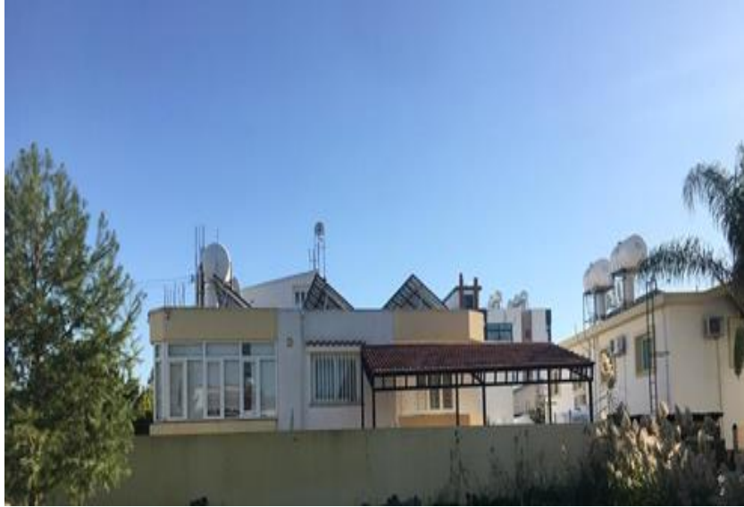
Figure 18: West facade (Author, N.U)
