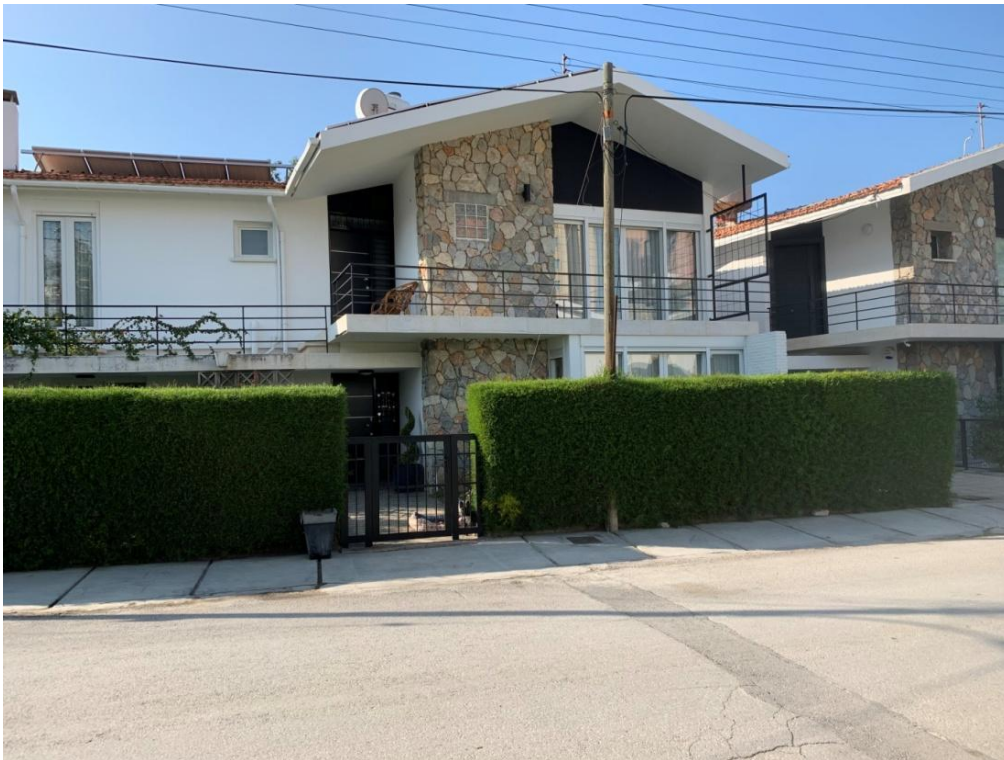
Figure 14: The front facade, partially covered with exposed local stone (Author, N.U).
