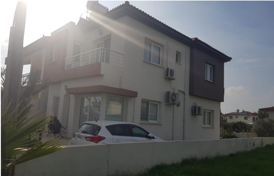
Figure 20: Front facade facing East (Author, N.U)
