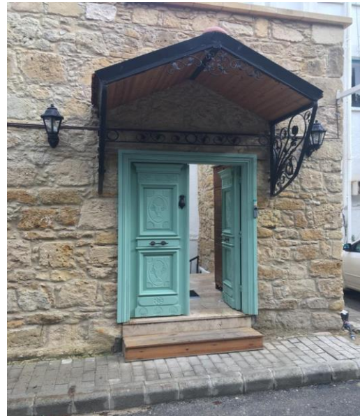
Figure 4. The historical and contemporary elements add a special style to the buildings (Author N.U.)
