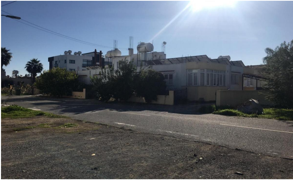
Figure 16: Back of the house facing South (Author, N.U)
