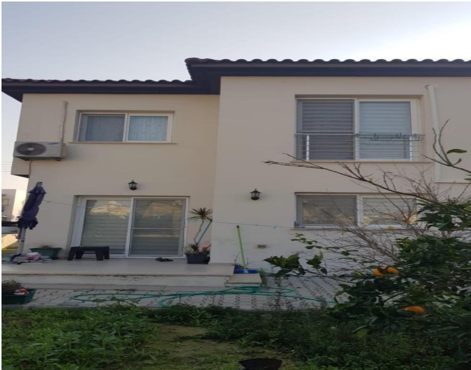
Figure 21: Back facade facing West (Author, N.U)
