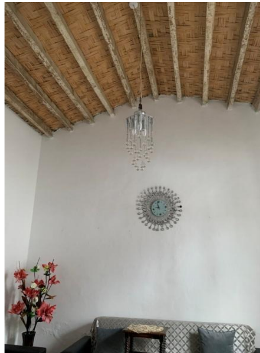
Figure 11: Room with a high ceiling covered with woven reed mats (Author N.U)
