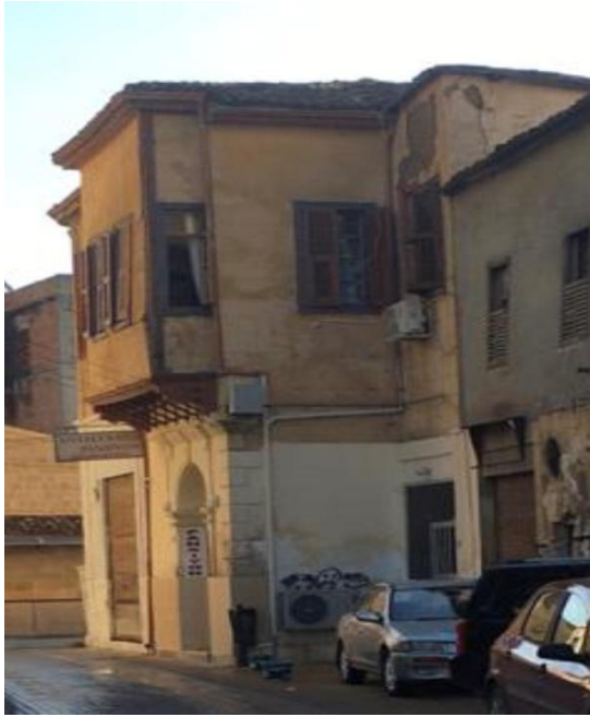
Figure 1. Stone on the ground floor wall adobe on the first floor walls of Ottoman house with bay window (Author, N.U)
