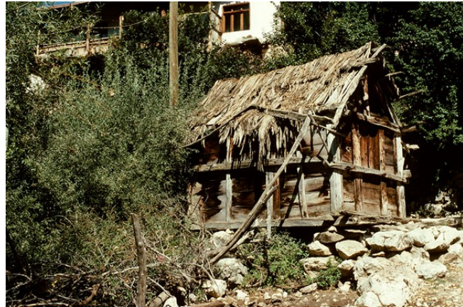
Fig. 17. Before the Use of tile and Metal Sheet Cover on the Roof Formed by the Wooden Timbers Called Harlama, Juniper Bark, Stems and Leaves of Corn and Reeds were Also Used as a Protective Upper Cover
