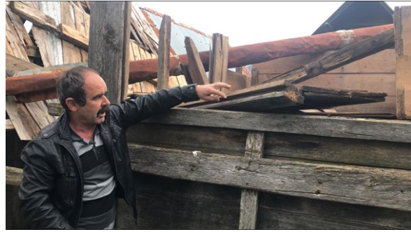
Fig. 16. Muhsin Ok, the Last Granary Craftsman, Shows the 2 cm Wide Keniş Section Opened on the Plank, the Fixing Plank Placed Vertically on the Wooden Piles is Called Morsa
