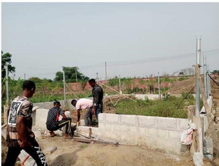
Figure 2. A typical building construction site.
