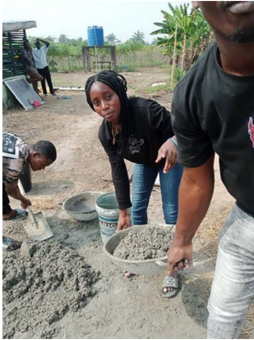
Figure 4. Taking of fresh concrete for laboratory analysis.
