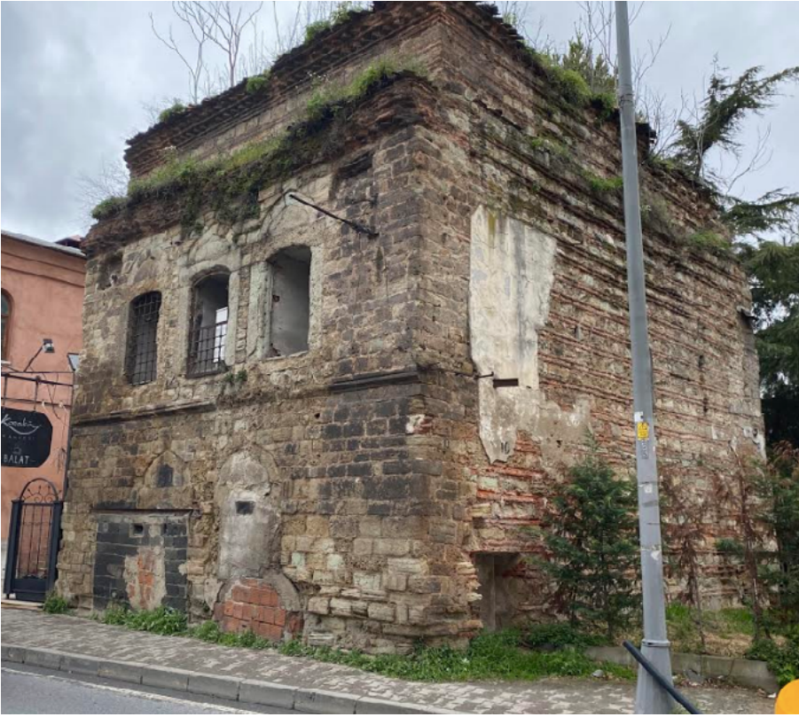
Figure 20: A small scale Phanar masonry wing with double hedgehog cornice. Photograph: Firuzan Melike Sümertaş, 2022.
