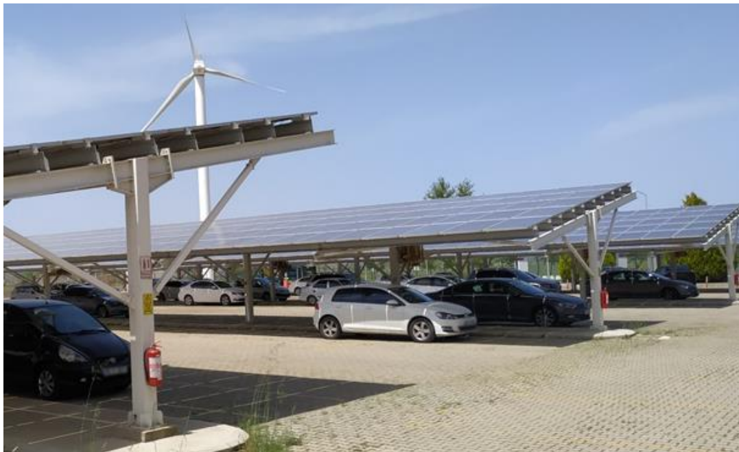
Figure 3. SPP installed on the steel construction in the parking lot.
