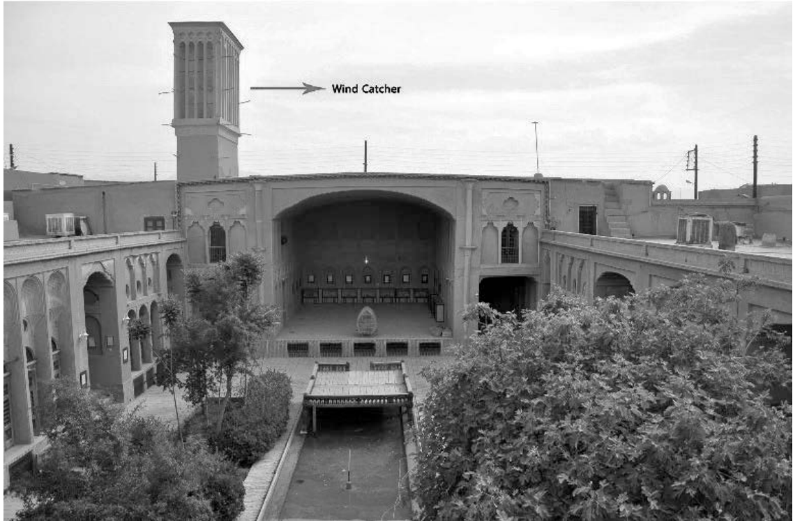
Figure 20. Wind catcher on the roof of Lariha house.
