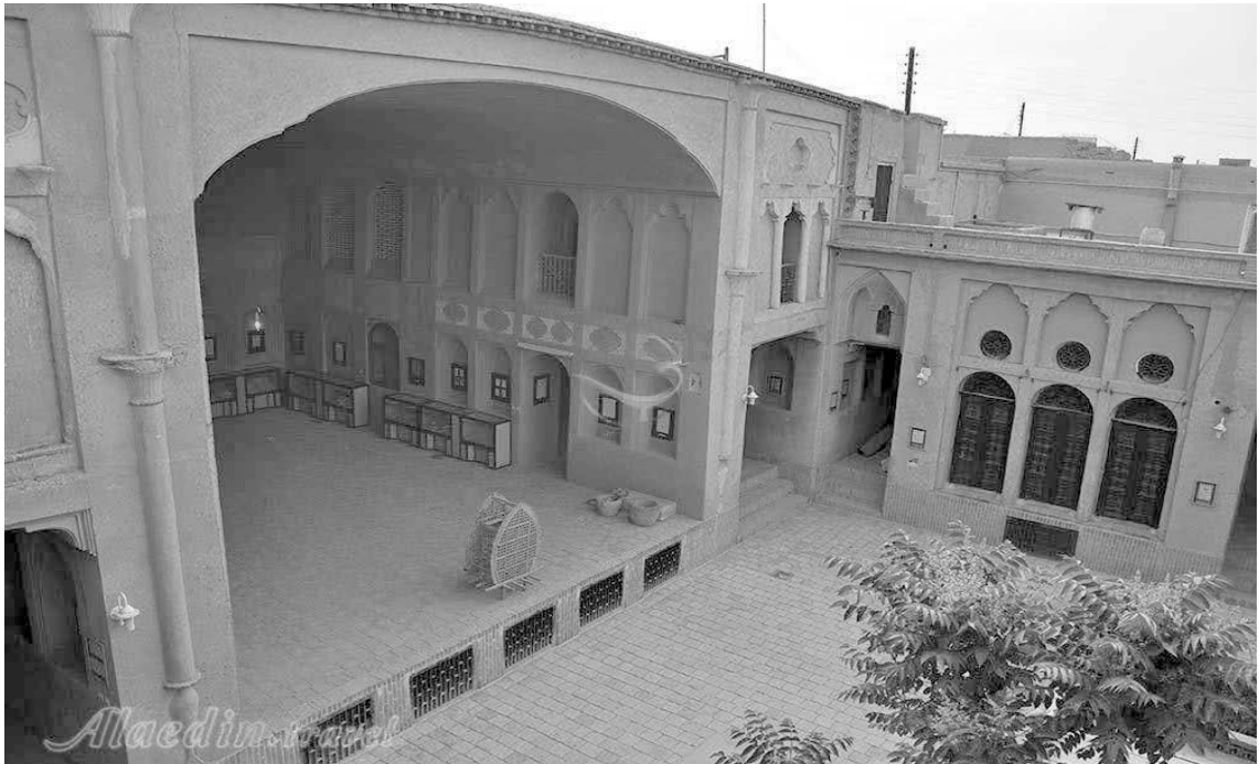
Figure 17. The large porch of the Lariha house
