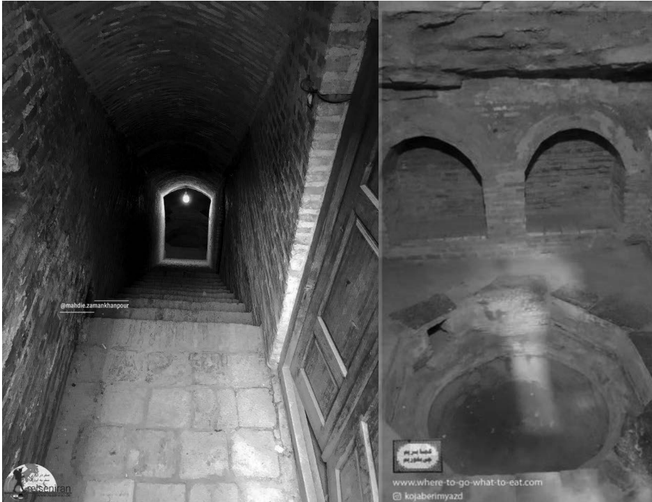
Figure 21. Sardaab (Water cellar) of Lariha houses
