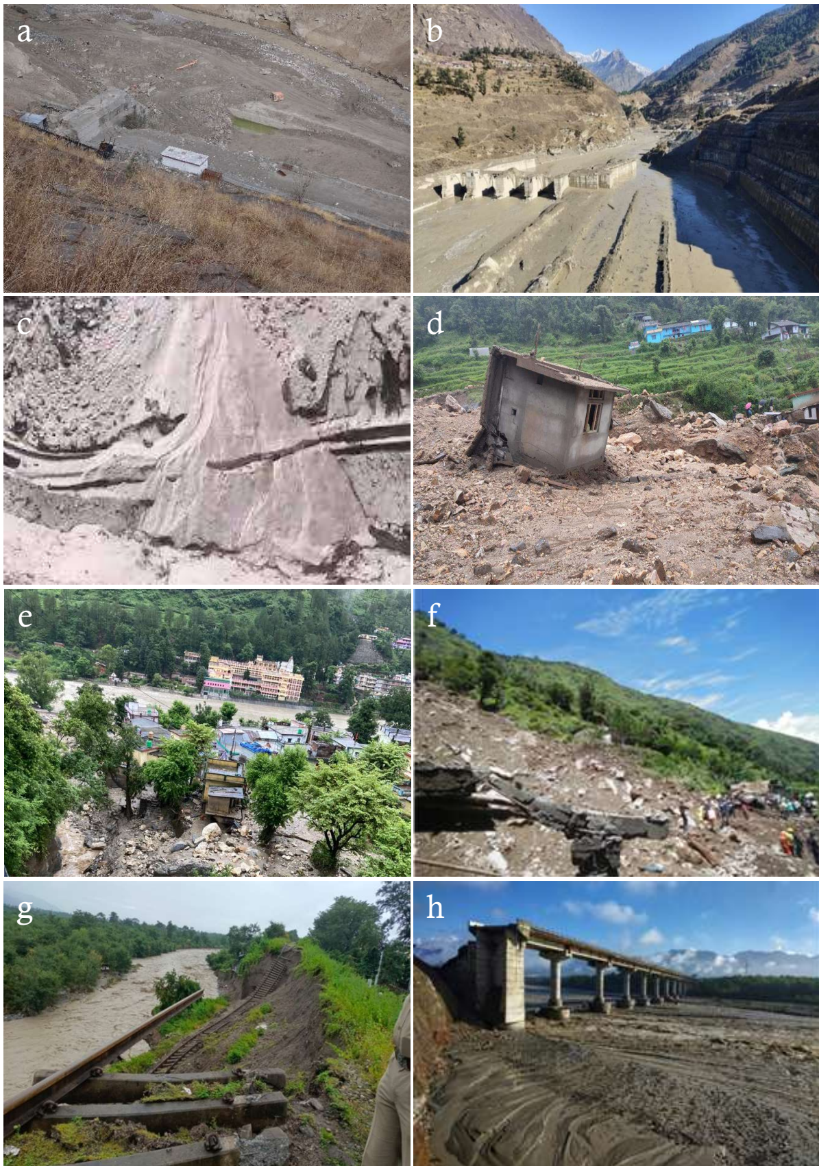
Fig. 4. Rock fall, flash flood/flood, avalanche and heavy localised rains or cloudbursts associated damages (a) washed away Rishiganga hydro project, (b) badly damaged Tapovan-Vishnugad hydro project, (c) an avalanche triggered near Sumna, (d) Ruined a house at Kankarari Village, (e) property damages in Mando Village, (f) damaged house at Jumma, (g) eroded railway track between Kathgodam and Haldwani and (h) damaged Gaula Bridge in Haldwani
