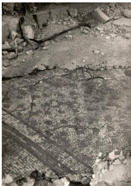
Figure 10 In situ the mosaic floor of the bema and apse, looking northeast (archives file no. 15/1962, courtesy of IAA).
