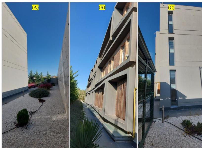
**Figure 2.** The examples of problem definition of distances that restrict photogrammetric techniques between the building and the surrounding wall (A: Side Facade, B: Back Facade, C: Side Facade)
