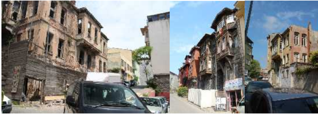
Figure 6: Views of dilapidation examples
