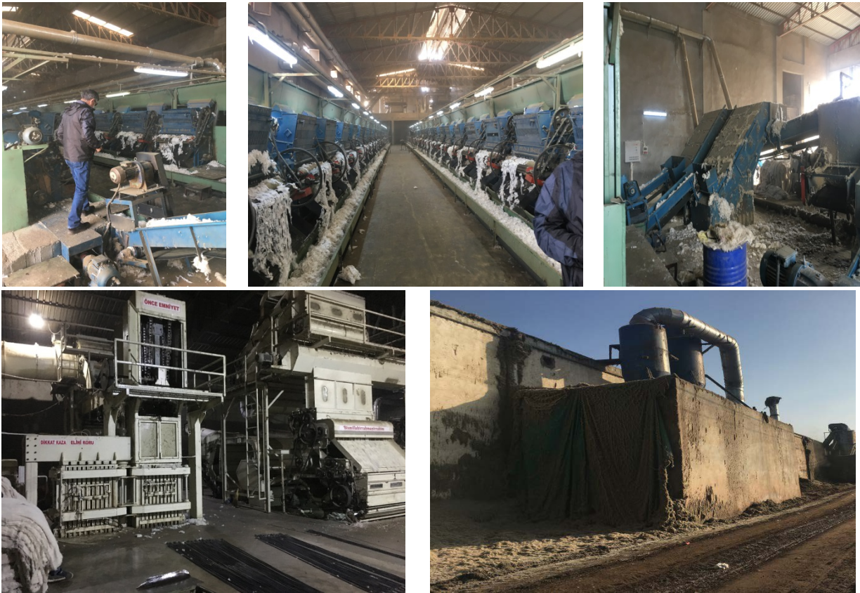
Figure 1. Some views of the ginning machines of factories
