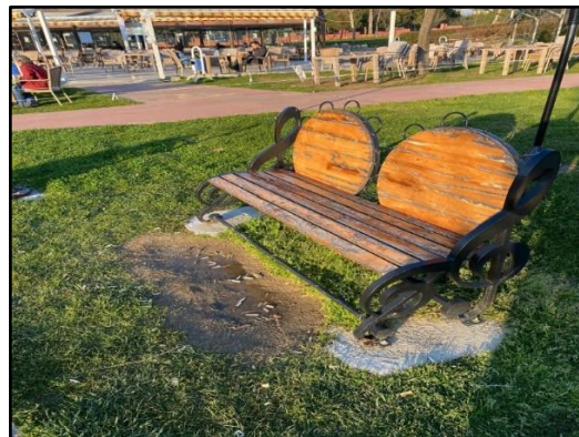
Figure 24. Sludge due to soil wear (Original, 2022)
