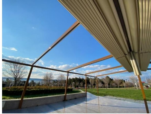
Figure 33. PVC tarpaulin shading element (Original, 2022)
