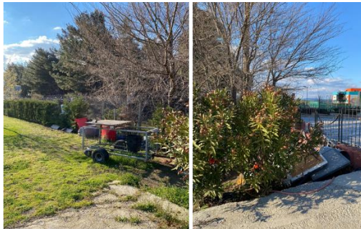
Figure 21. Stacked materials (Original, 2022)
