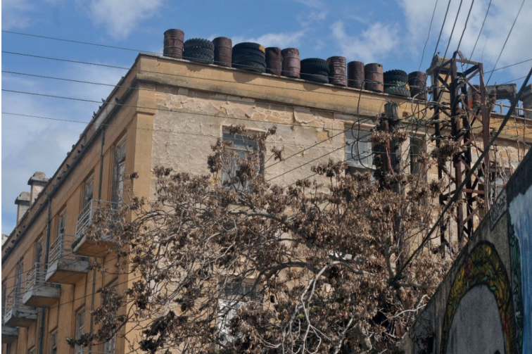
Photograph 4. The roof of an abandoned building covered with barrels from wartime.
