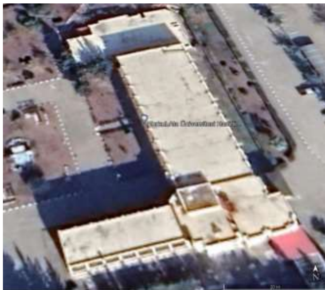
Figure 1. The location and satellite image of the building
