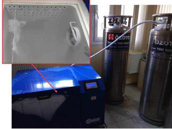
Şekil 4. PLC kontrollü kriyojenik tank (PLC controlled cryogenic tank)
