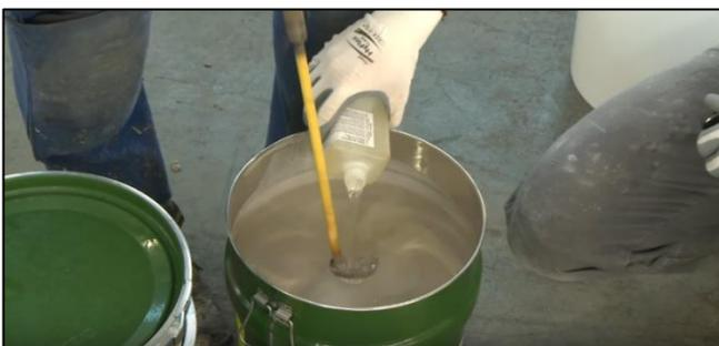
Figure 15. Mixing silicone & hardener component
