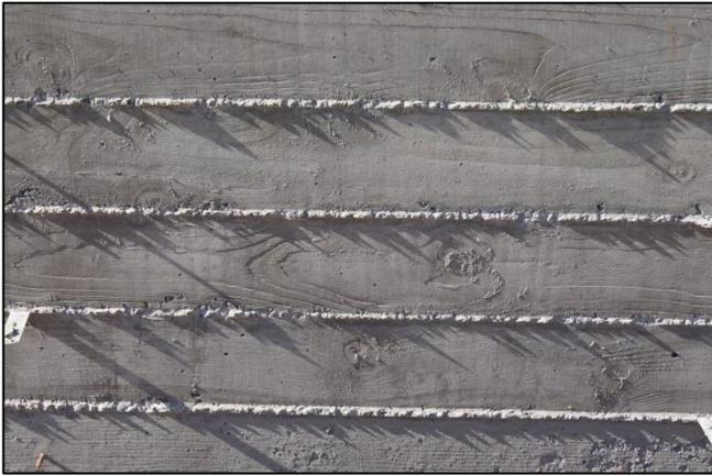
Figure 1. Mold board prints on concrete surface.
