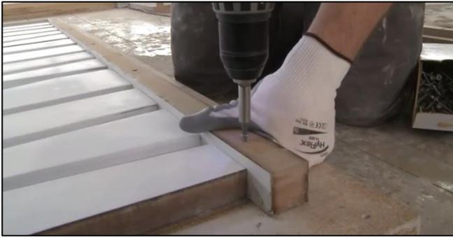
Figure 12. Assembling molding frame
