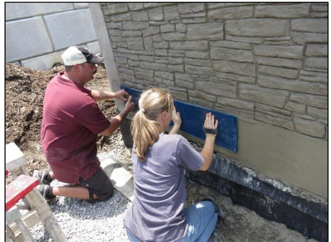
Figure 4. Stamping method on concrete surface
