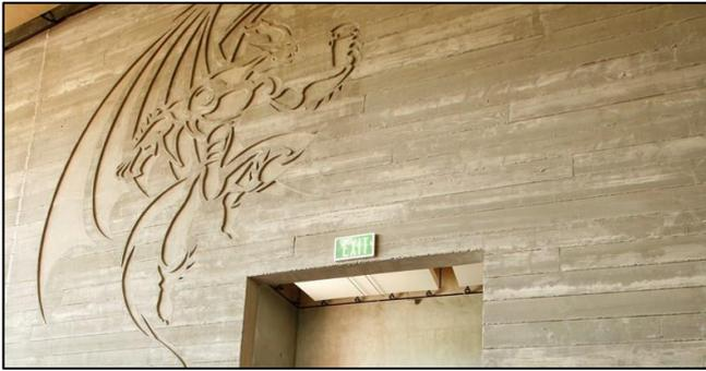
Figure 6. Negative patterns on concrete surfaces
