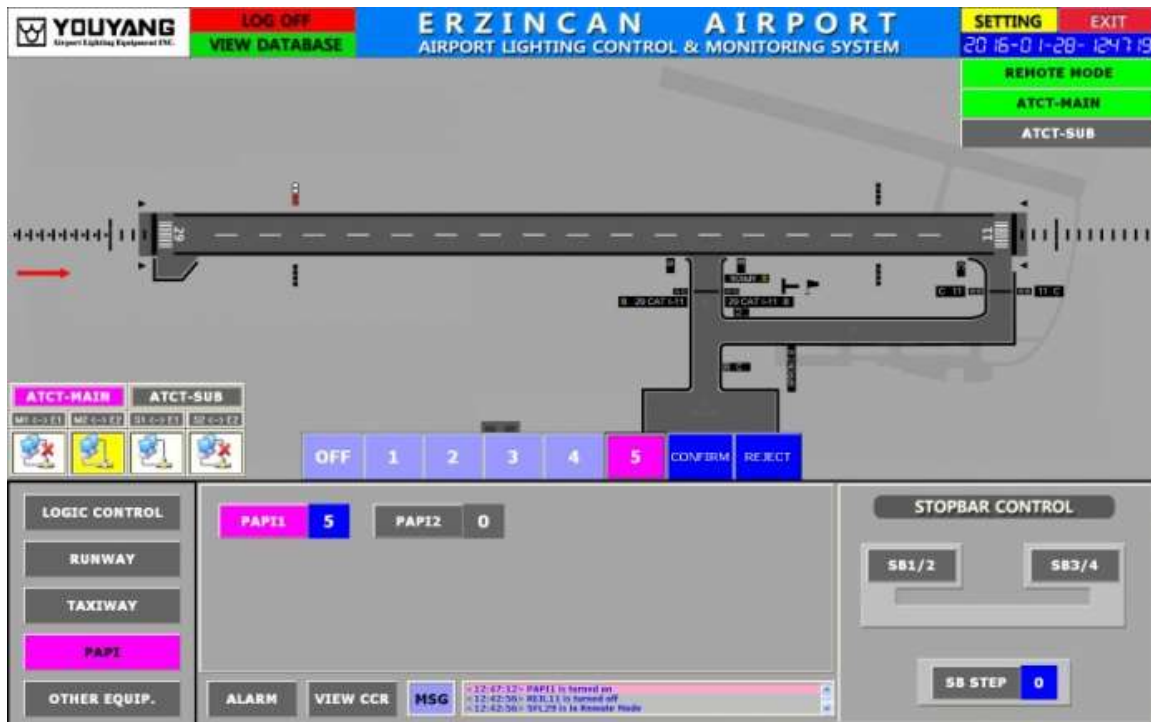
Figure 19. Commissioning of the PAPI system using the control screen
