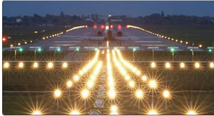
Figure 8. Runway Centre-line light [14]
